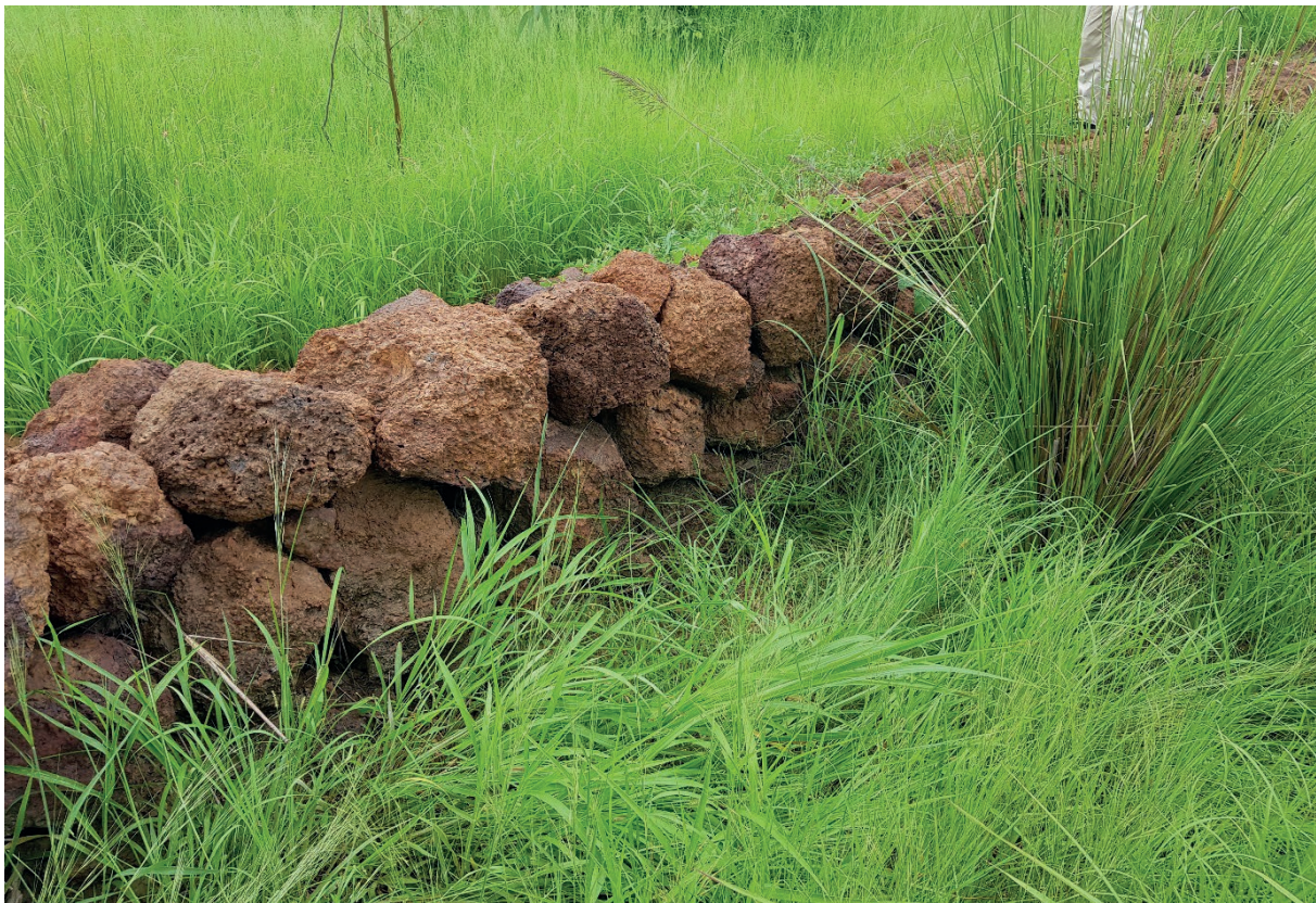
Photo 4: Filtering dyke
